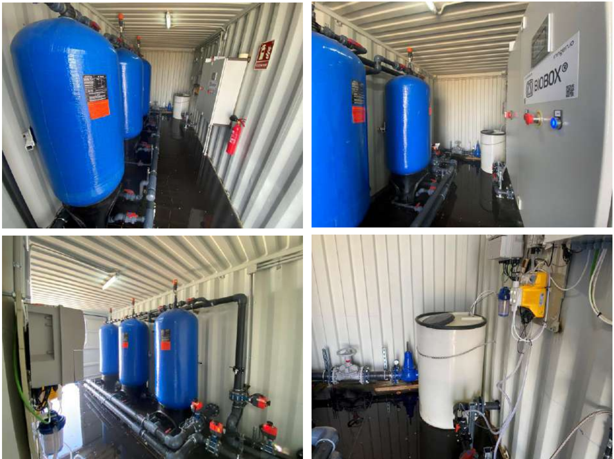
Figure 2: Photos of the interior of the BIOBOX Turbidity 15m 3 /h plant
