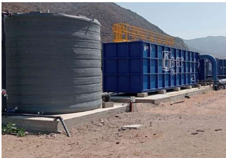
Figure 1: BIOBOX Ammonium Plant 44-52 GPM /10-12 m 3 /h
